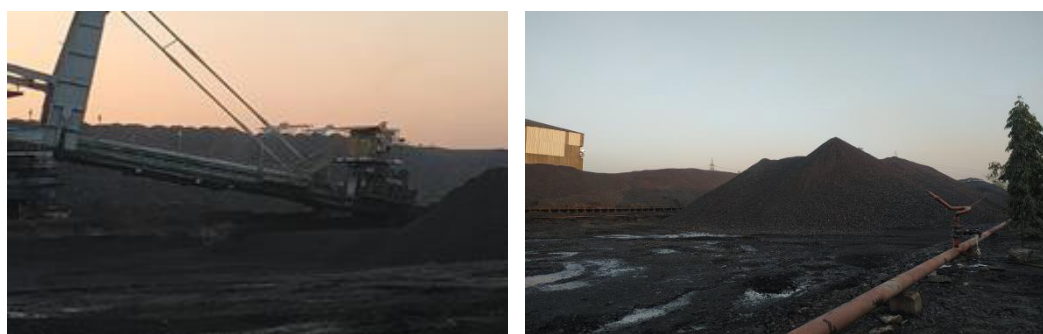
Figure 4.1: Coal handling area at the stackyard
